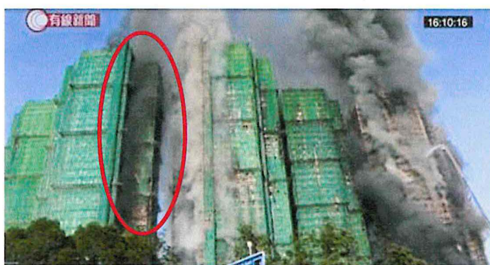
Pyrolyzed gases from combustibles accumulated in the re-entrant 11
