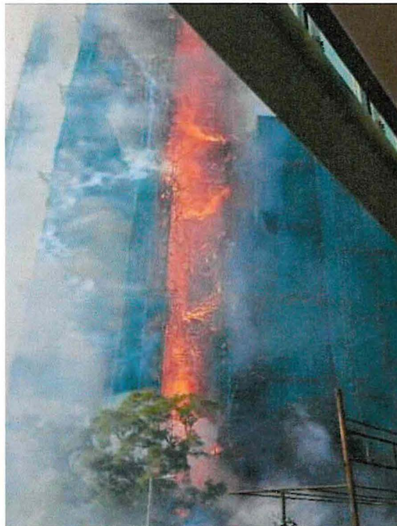
Rapid vertical fire spread observed at Wang Cheong House
