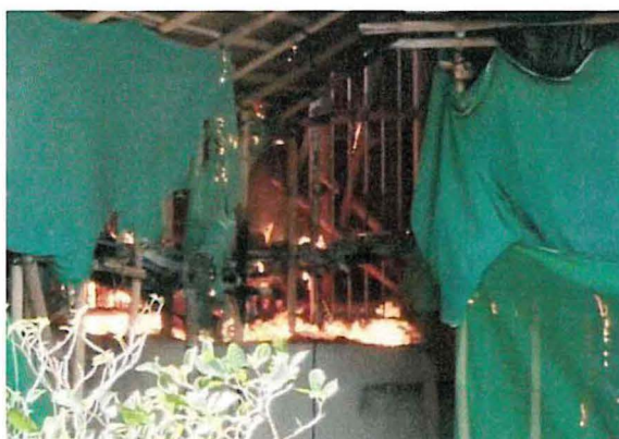
Incipient stage of the fire on the flat roof outside Rooms 104 and 105 of Wang Cheong House
