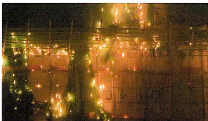
Falling fragments of burning scaffolding nets contributing to fire spread
