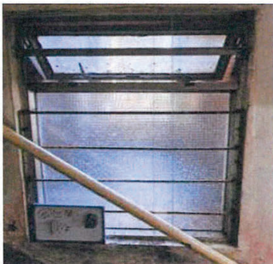
Photo 1(c): Staircase Window (Before renovation works)
