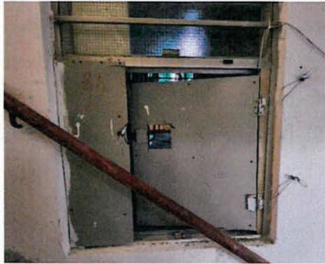
Photos 2 (a) & (b): Replacement of Windows with Movable Boards
