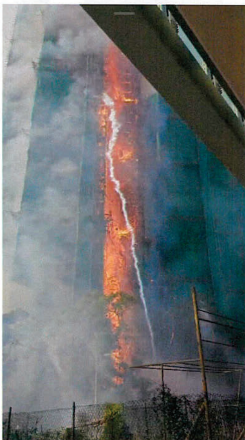
Photos 4 (a) to (c): Fire Intensified and Engulfed the Entire East Re-entrant of Wang Cheong House with Falling Debris at 1458 hours
