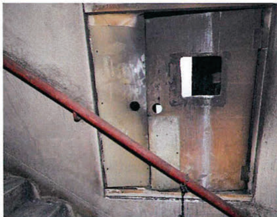
Rear Staircase between 25/F & 26/F
