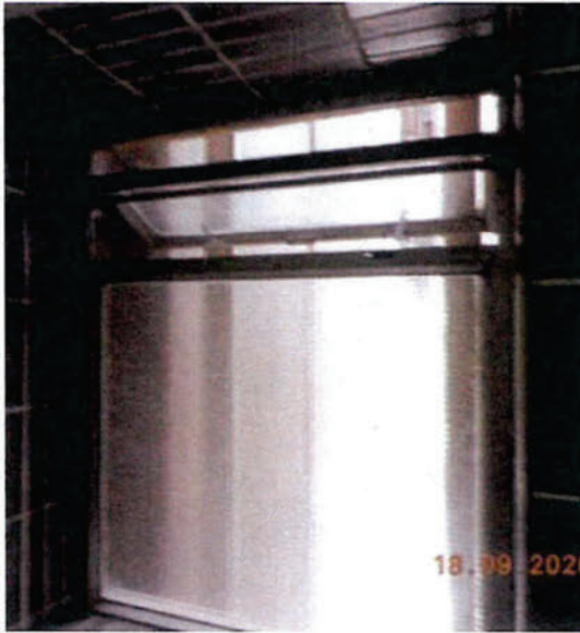
Photo 1 (a): Lift Lobby Window (Before renovation works)
