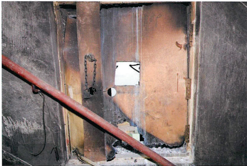
Photos 2 (a) & (b): Replacement of Windows with Movable Boards
