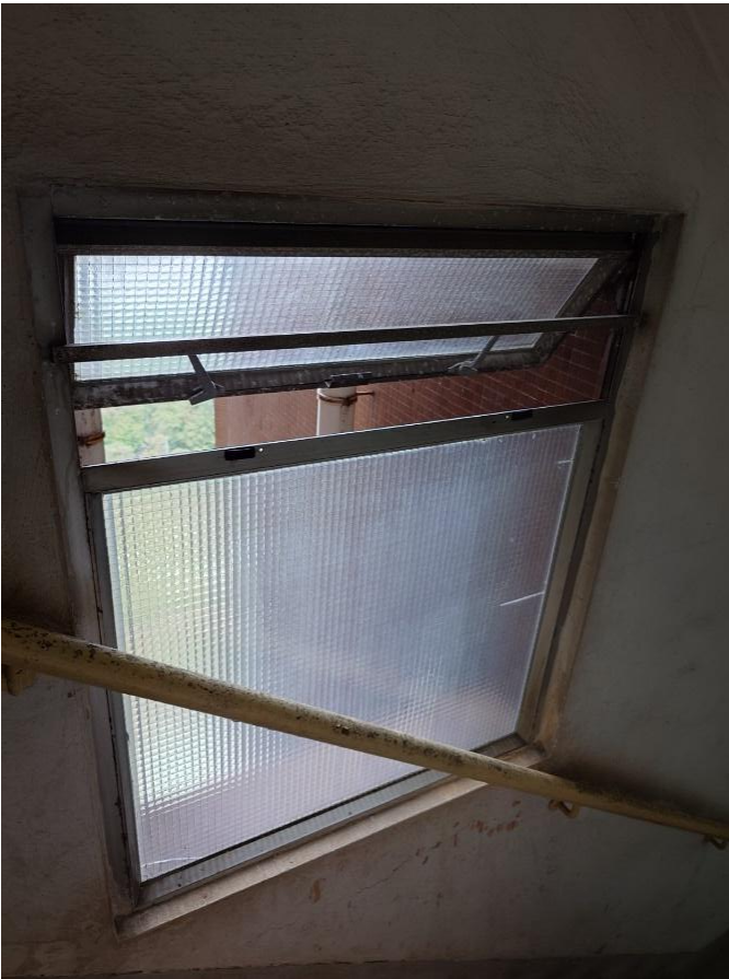
Figure 4.7. Wired glass window (WG) in (a) staircase; (b) lift lobby
