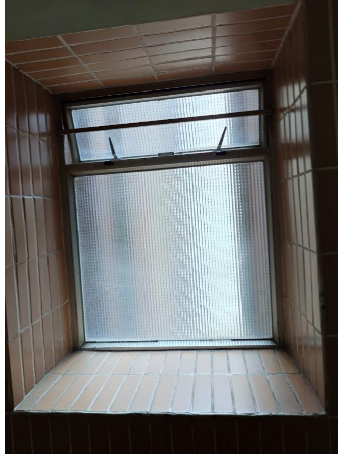
Figure 4.7. Wired glass window (WG) in (a) staircase; (b) lift lobby
