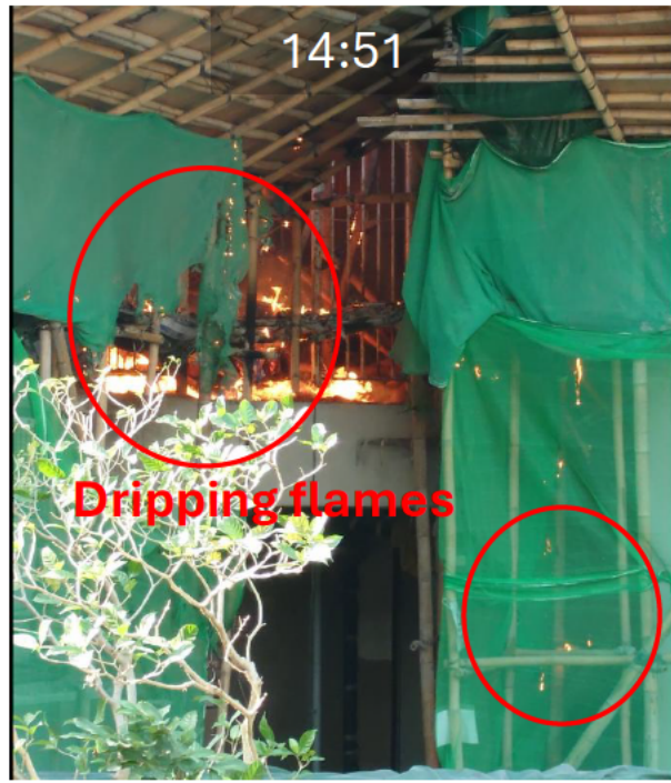
Initiation of fire at flat roof
