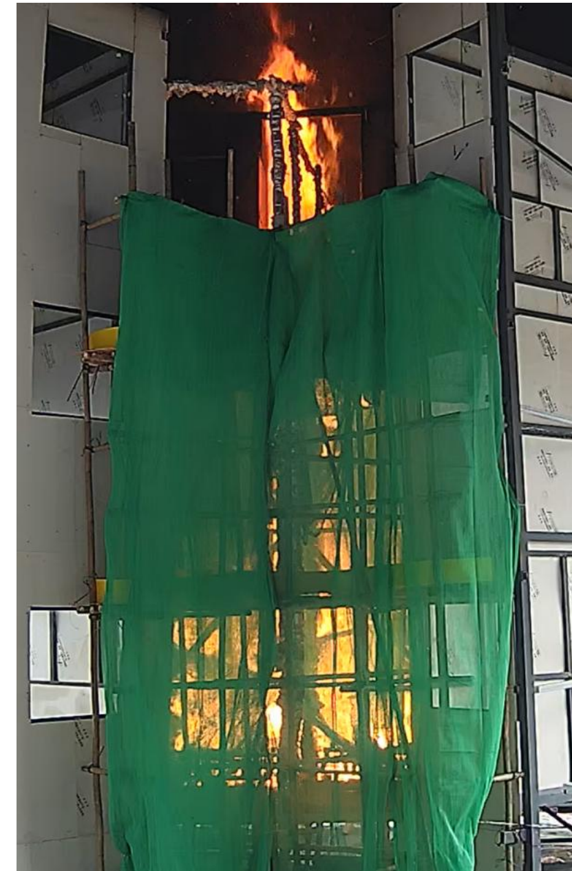
Full Developed Fire in Test 4 using FR Safety Nets
