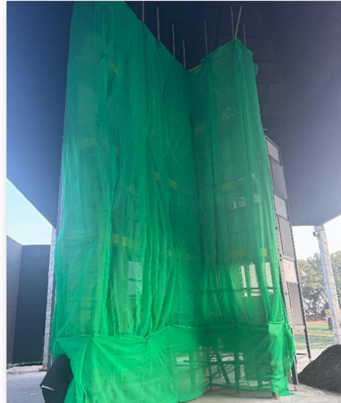
External View With Safety Net
