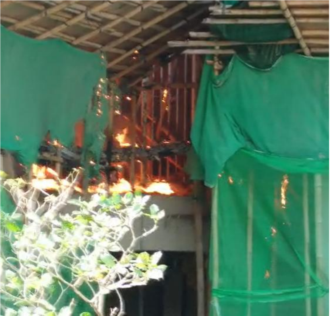
Front View: Re-entrant of Wang Cheong House
