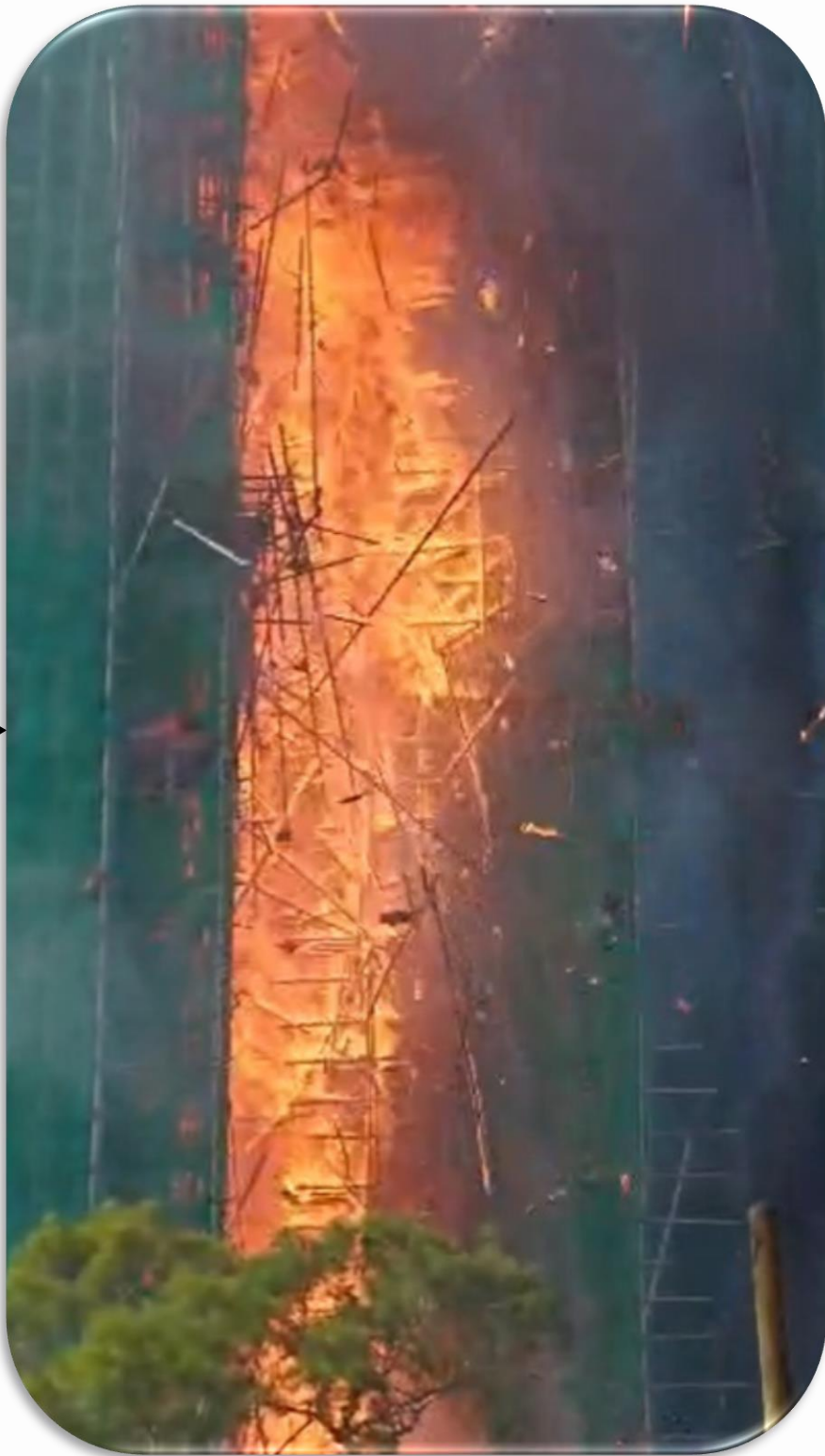
Rapid Vertical Fire Spread Along Re-entrant
