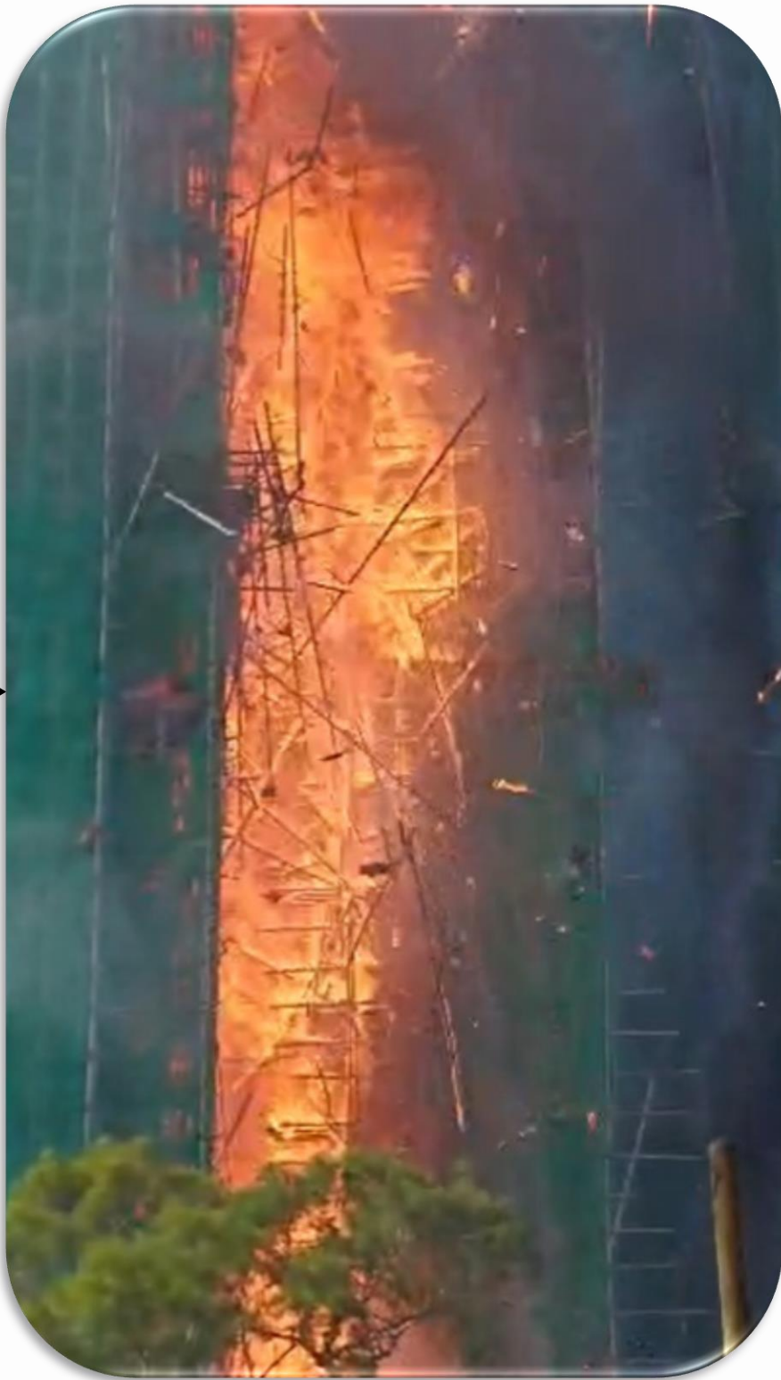
Rapid Vertical Fire Spread Along Re-entrant
