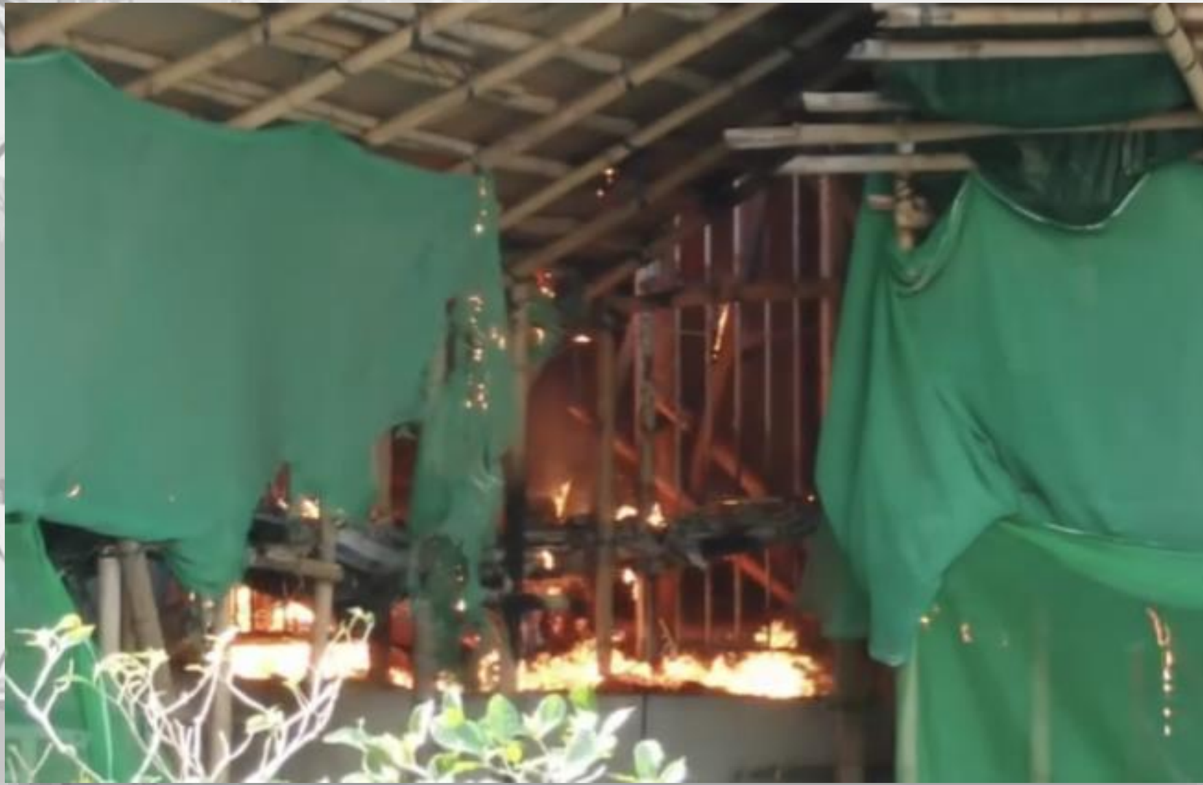
Discovery of Fire at Wang Cheong House
