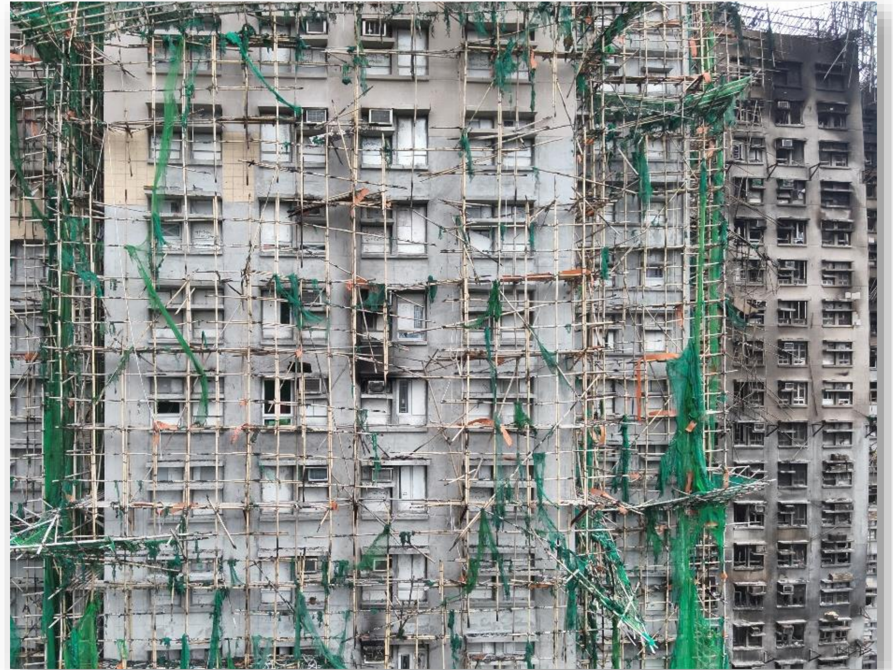
External View of Wang Kin House
