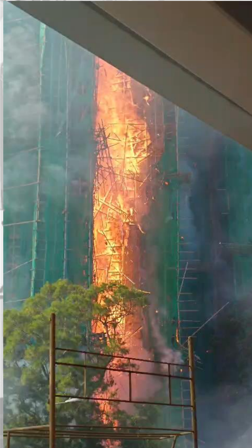
Wang Cheong House East Re-entrant 1458 Hrs
