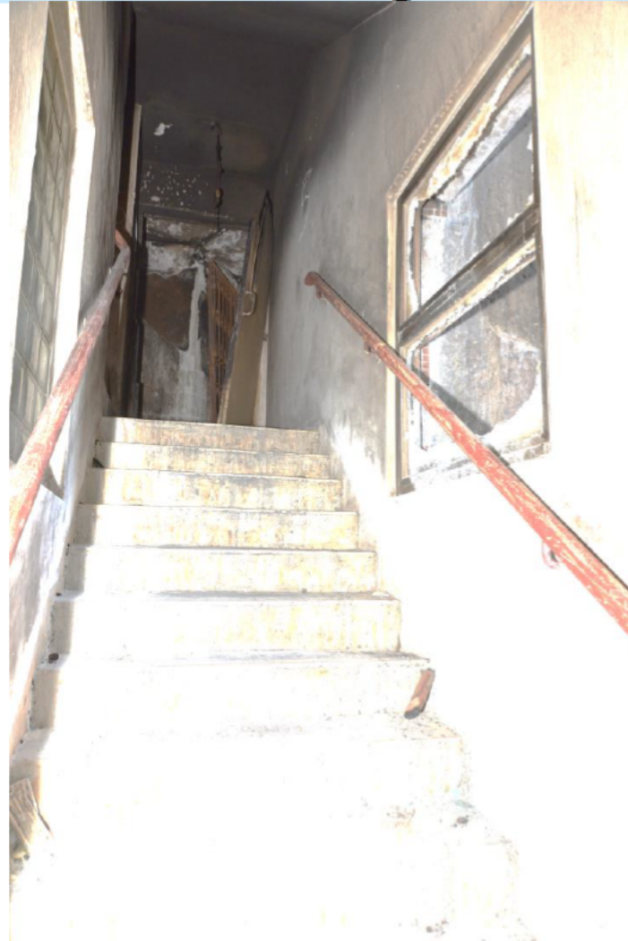
View of front staircase from 4/F to 5/F
