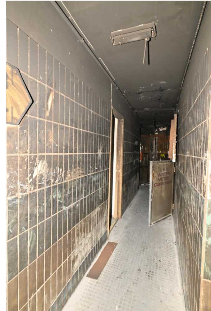
View of corridor from Flat 101-102 towards Flat 103-104, with close-up view of the end of Flat 103-104 at Photo 2B
