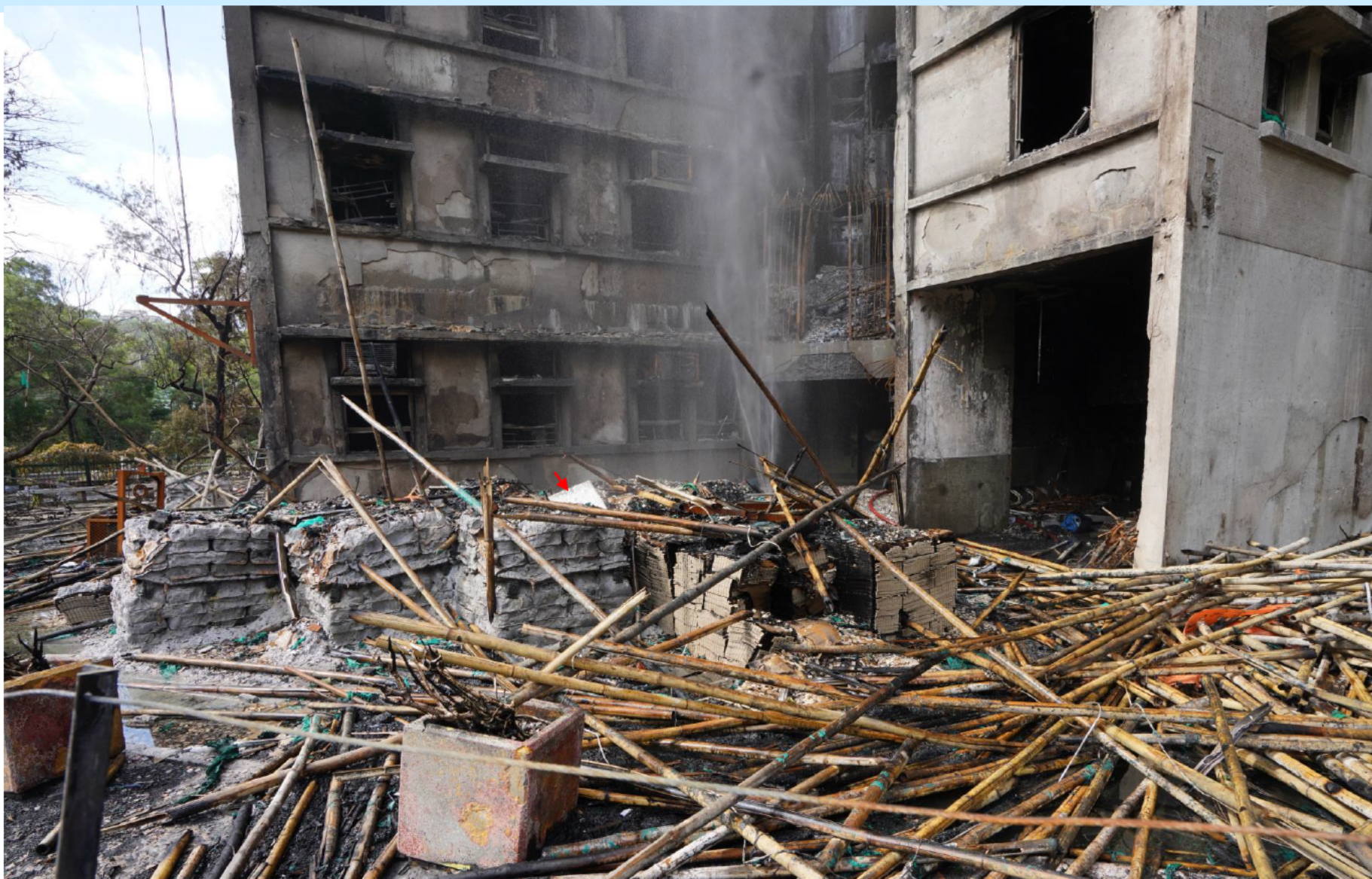
Photo 12: Outside the ground floor of side 4-5 of Wang Cheong House (collapsed scaffolds, such as burnt bamboo remains, remnants of safety nets and foam boards (↑) , with bags of plastering materials (with close-up at Photo 12a below) and carton paper boxes of mosaic tiles (with close-up at Photo 12b below) .
