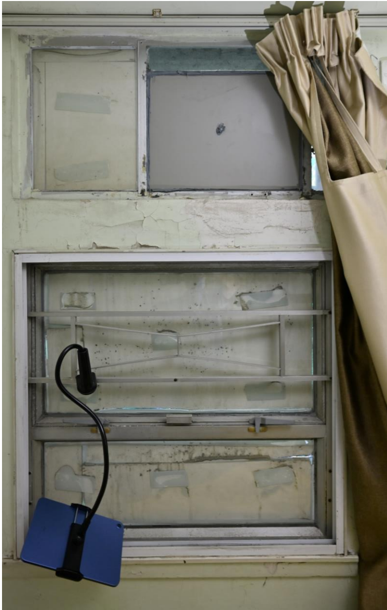
Wang Chi House, Room 03 bedroom
