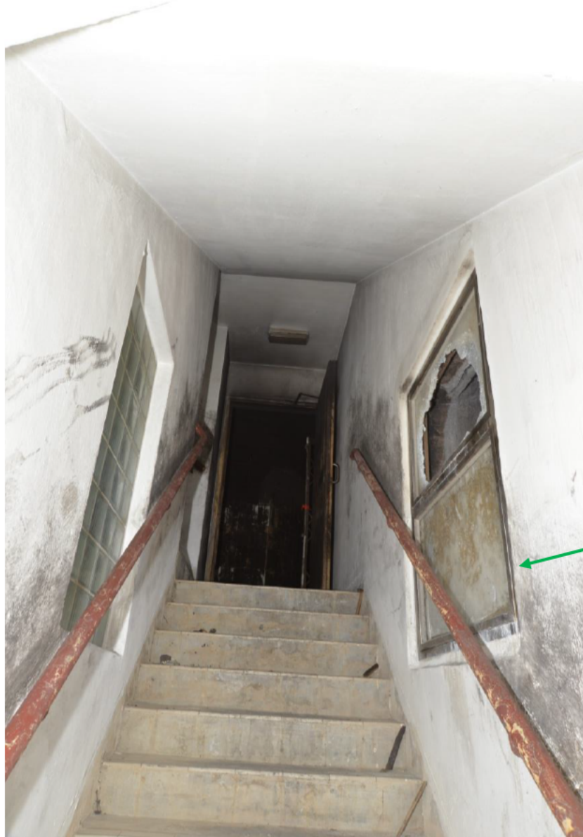
View of rear staircase from 3/F to 4/F
