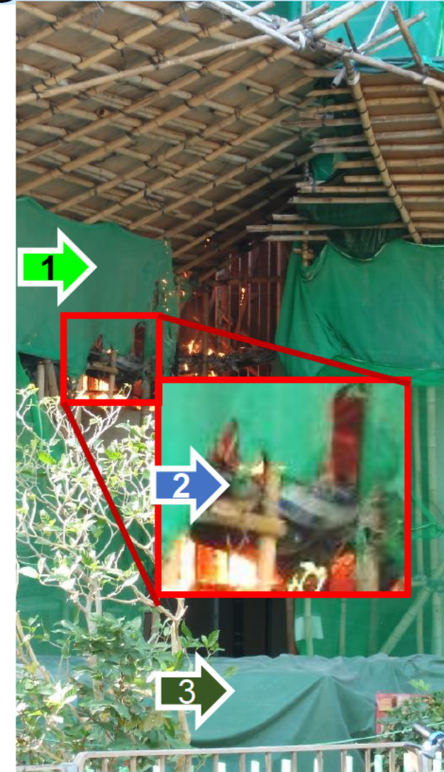
(3) Green plastic sheeting
