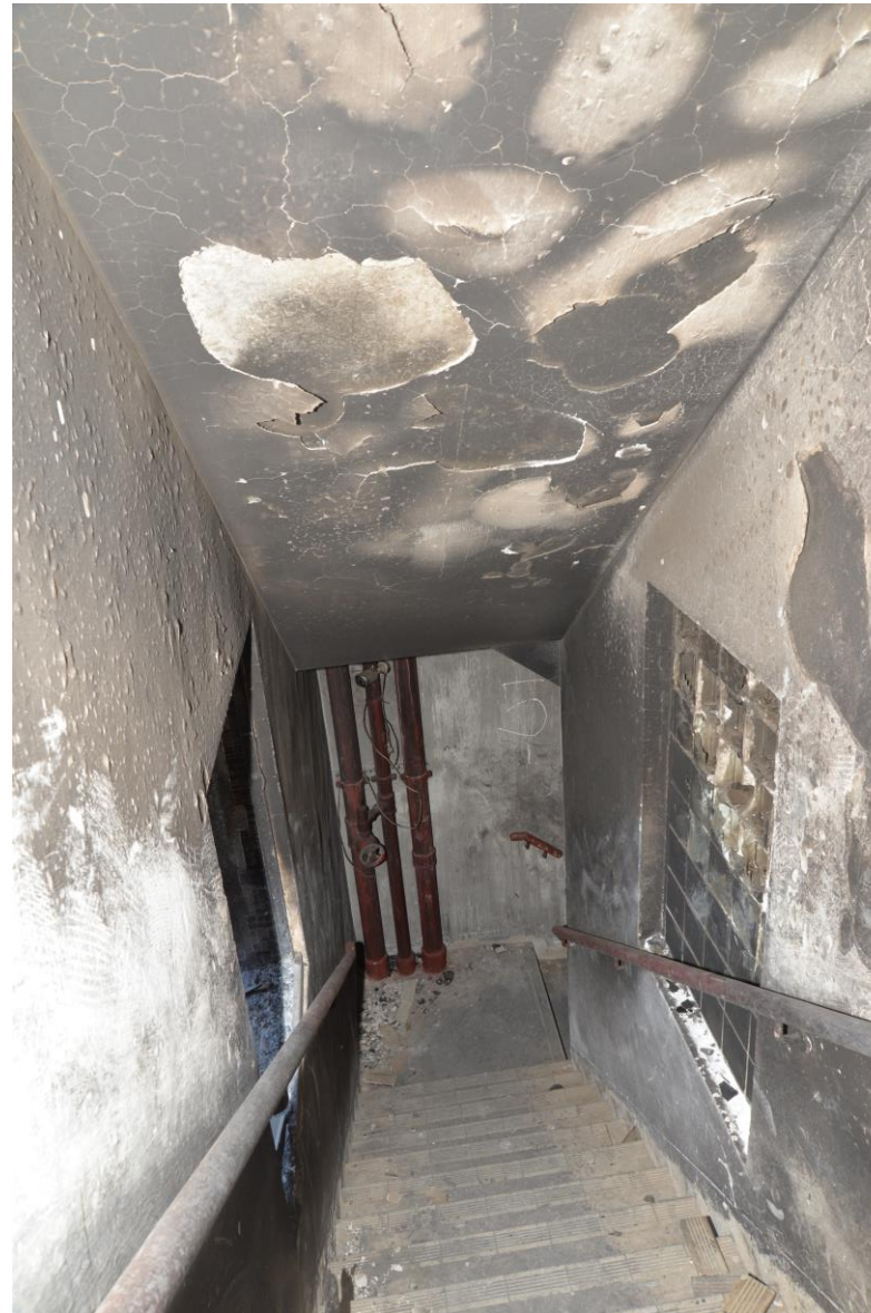
View of rear staircase from 5/F to 6/F, the window towards Light Well 4-5 had been removed leaving an intact wooden slat at the base of the opening. Severe heat damage above the opening
