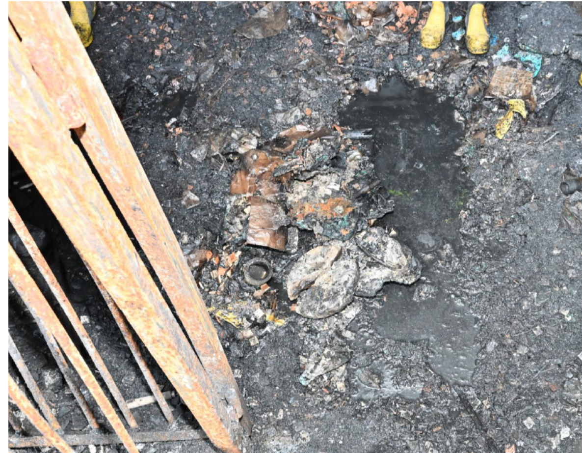
View of seat of fire from the metal gate
