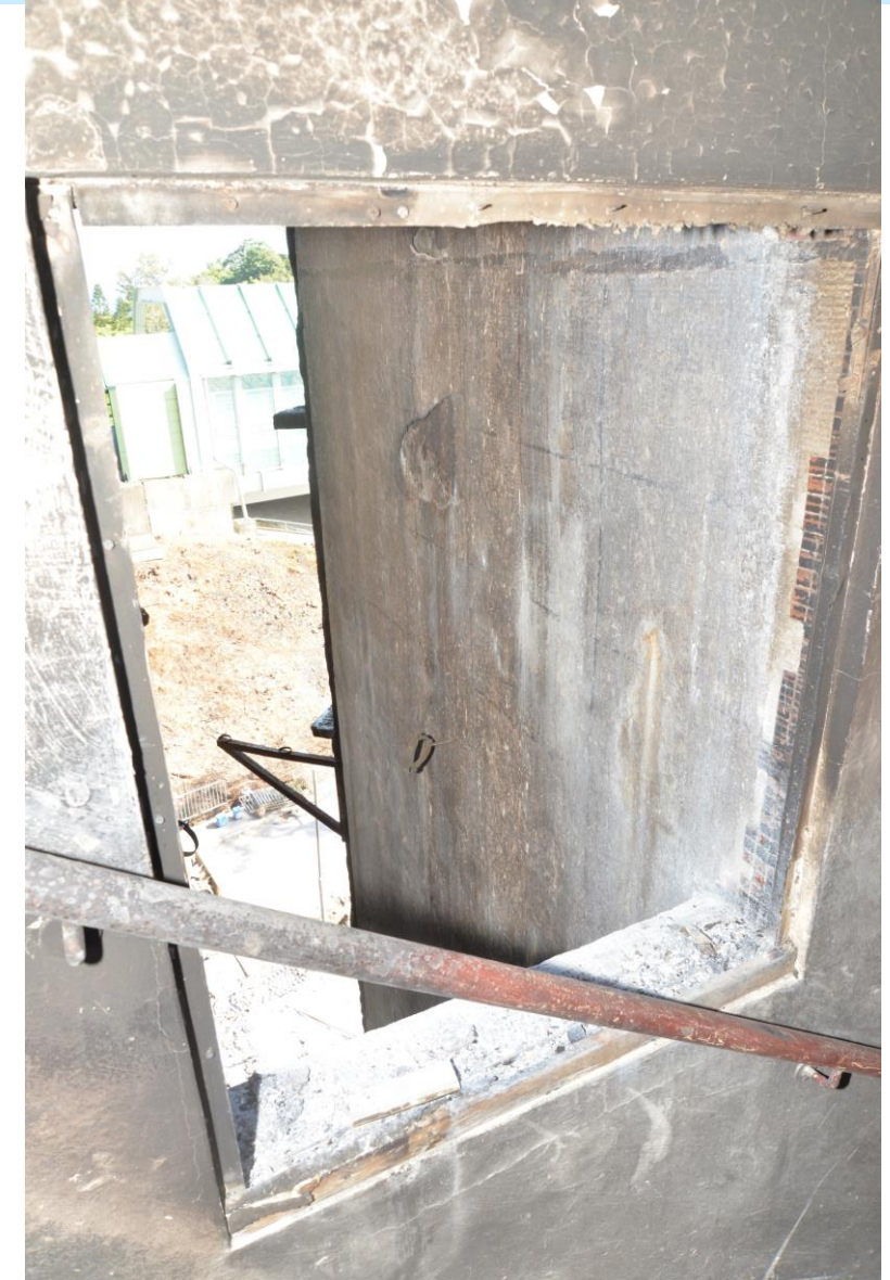
View of rear staircase from 5/F to 6/F, the window towards Light Well 4-5 had been removed leaving an intact wooden slat at the base of the opening. Severe heat damage above the opening
