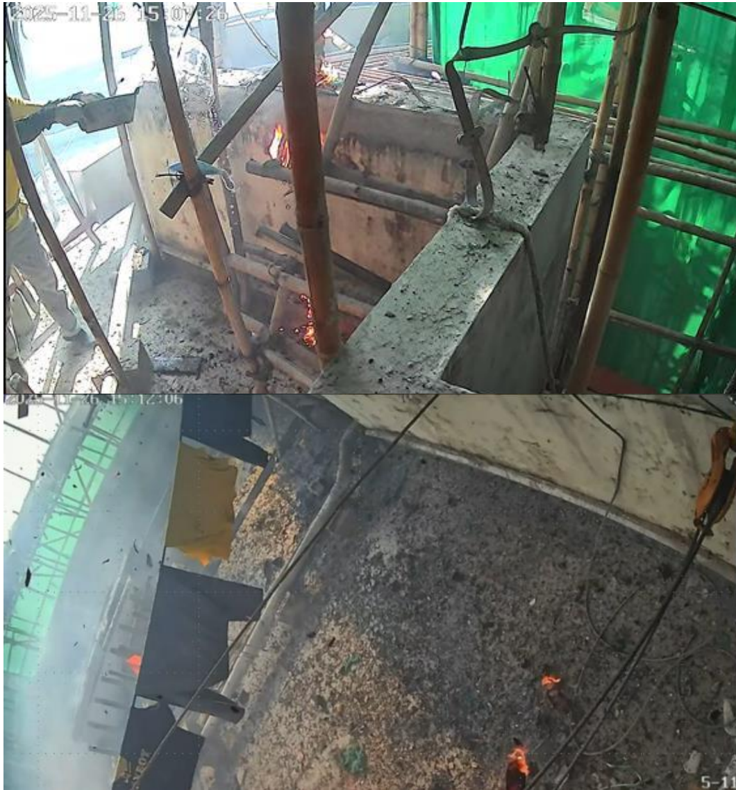
Photos 6-9 (a) & (b): Flying Embers Suspected Spreading from Wang Cheong House to Wang Tai House at about 1506 and 1511 hours 57
