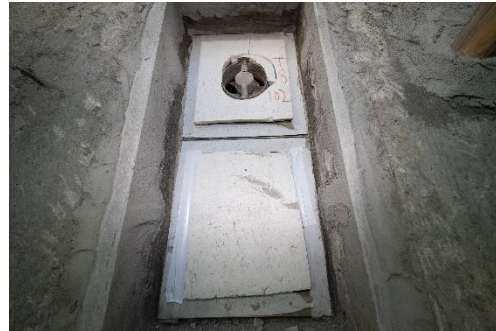
Photos 4-14 (a) to (c): Polystyrene Window Covers
