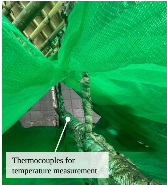
Photo 6-12 (e): Internal View with Safety Nets
