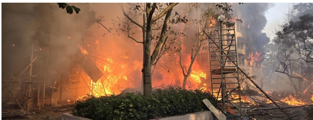
Photo 8-3: The Burning Debris and Bamboo Scaffolding Blocking Exits
