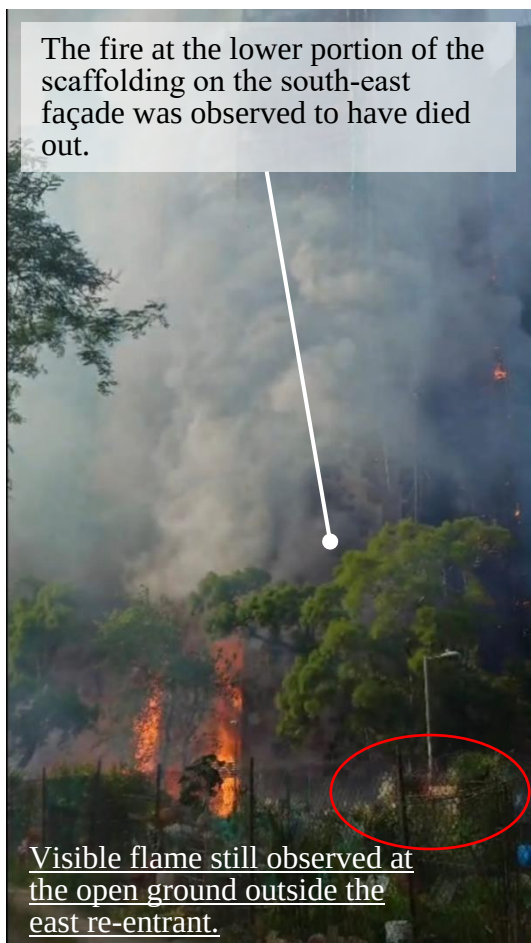
Photo 5-6 (c): Visible Flame still Observed at the Open Ground outside the East Re-entrant at 1508 hours
