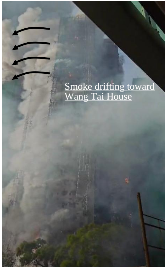
Photo 5-6 (e): Heavy Smoke on the South-east Façade at 1508 hours
