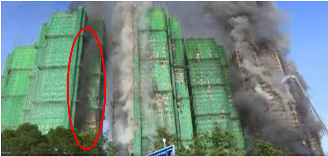
Photo 6-7 (c): Suspected Pyrolyzed Gases from Combustibles Accumulated in the Re-entrant
