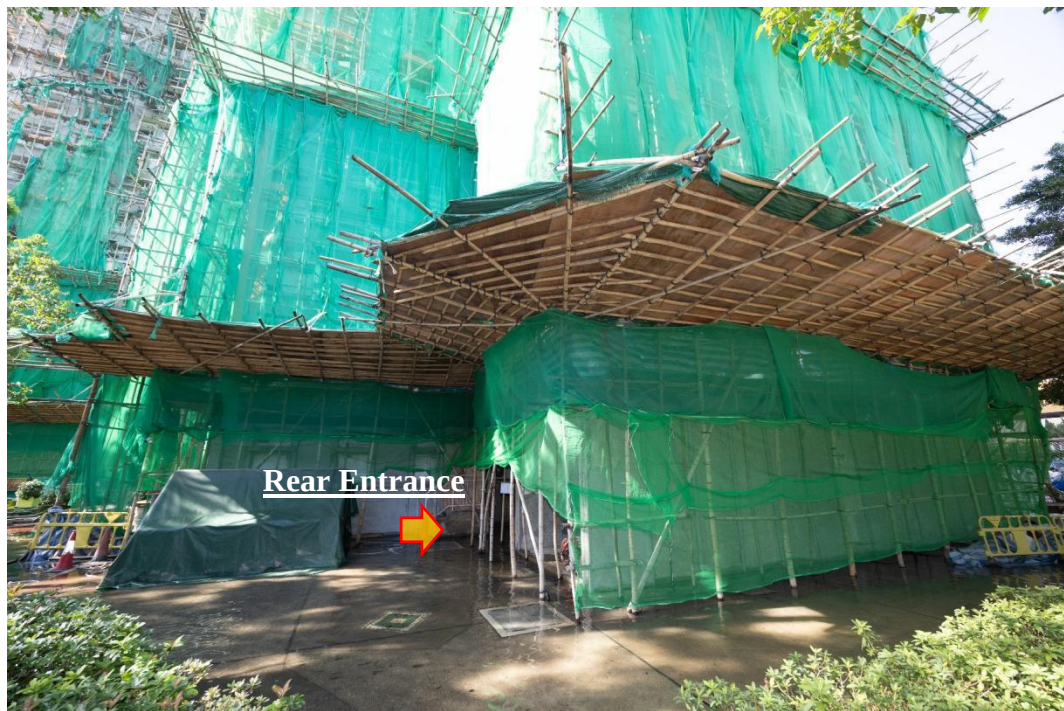
Photo 4-11 (b): Rear Entrance of Wang Chi House
