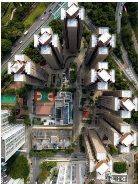
Photo 4-1: Wang Fuk Court (Photo taken in 2023) 5
