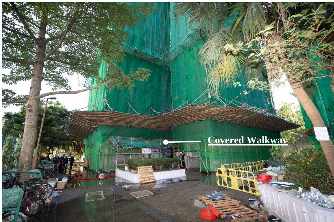
Photo 4-11 (a): Covered Walkway at the Main Entrance of Wang Chi House
