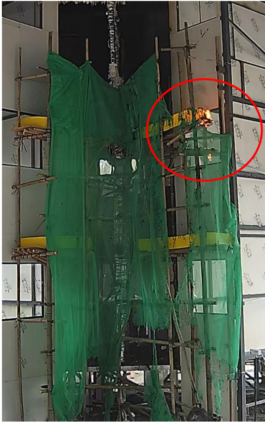
Photo 6-16 (a): Secondary Ignition Occurred in Test 3
