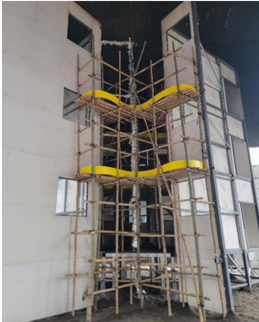
Photo 6-12 (b): Scaffolding Setup
