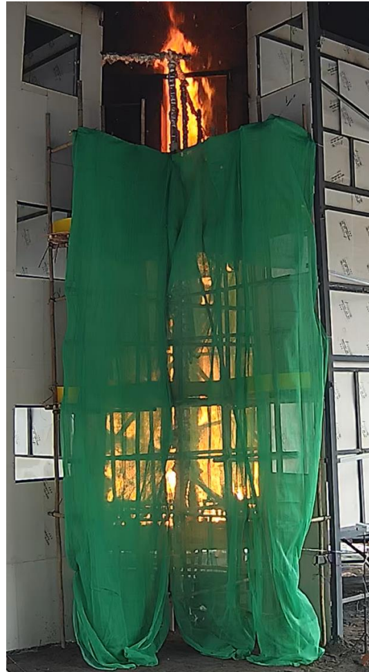
Photo 6-15 (b): Full Developed Fire in Test 4 (FR Safety Net)
