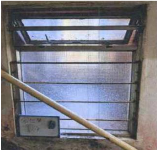
Photo 4-3 (a): Staircase Window (Before renovation works)
