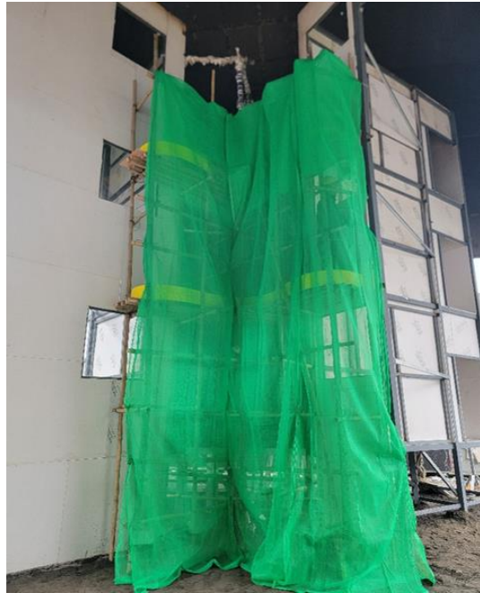
Photo 6-12 (c): External View with Safety Nets
