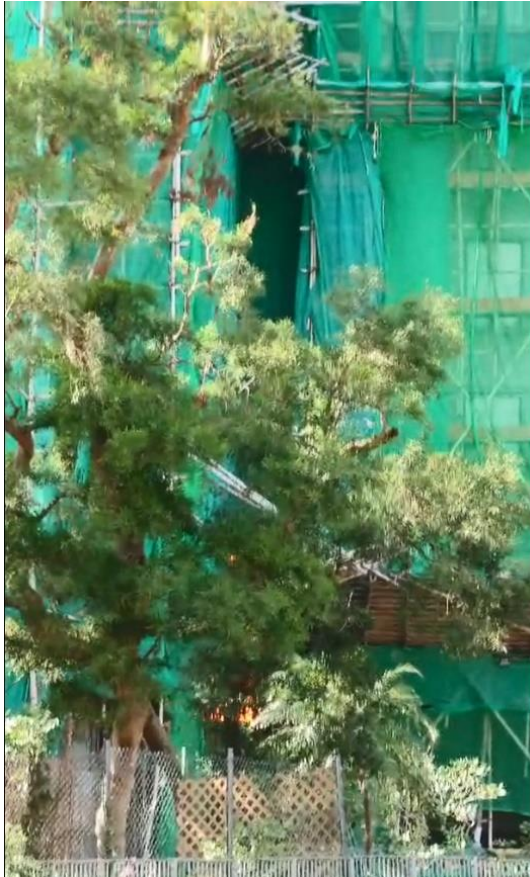
Photo 5-3: Fire Spread to about 4/F at about 1455 hours
