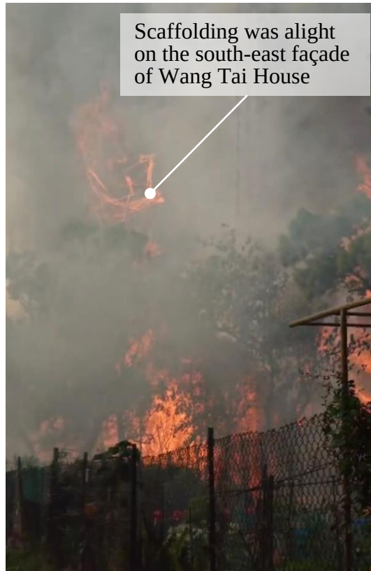
Photo 5-7 (b): South-east Façade of Wang Tai House Alight at 1515 hours
