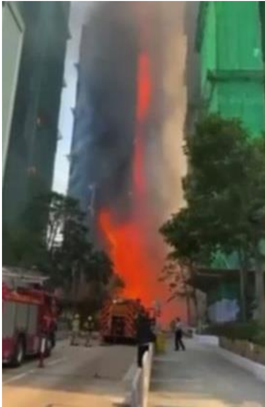
Photo 5-7 (a): Fire Spreading along the West Re- entrant at 1511 hours
