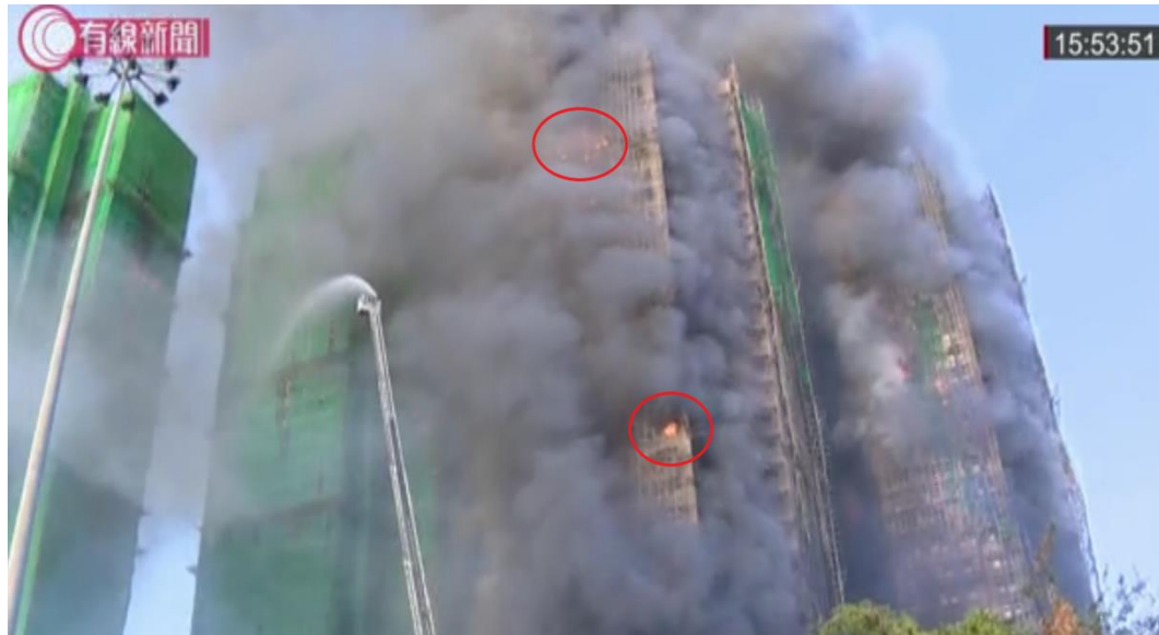
Photo 5-11: Flames from Ignited Units on the South-west Façade of Wang Tai House
