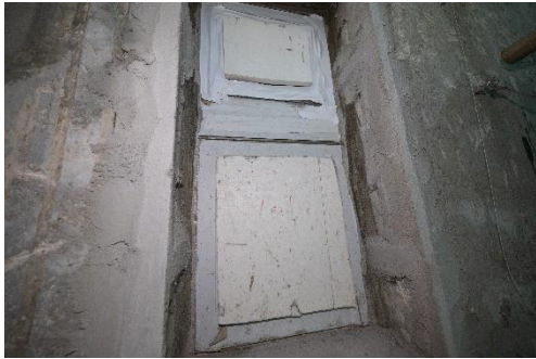
Photos 4-14 (a) to (c): Polystyrene Window Covers
