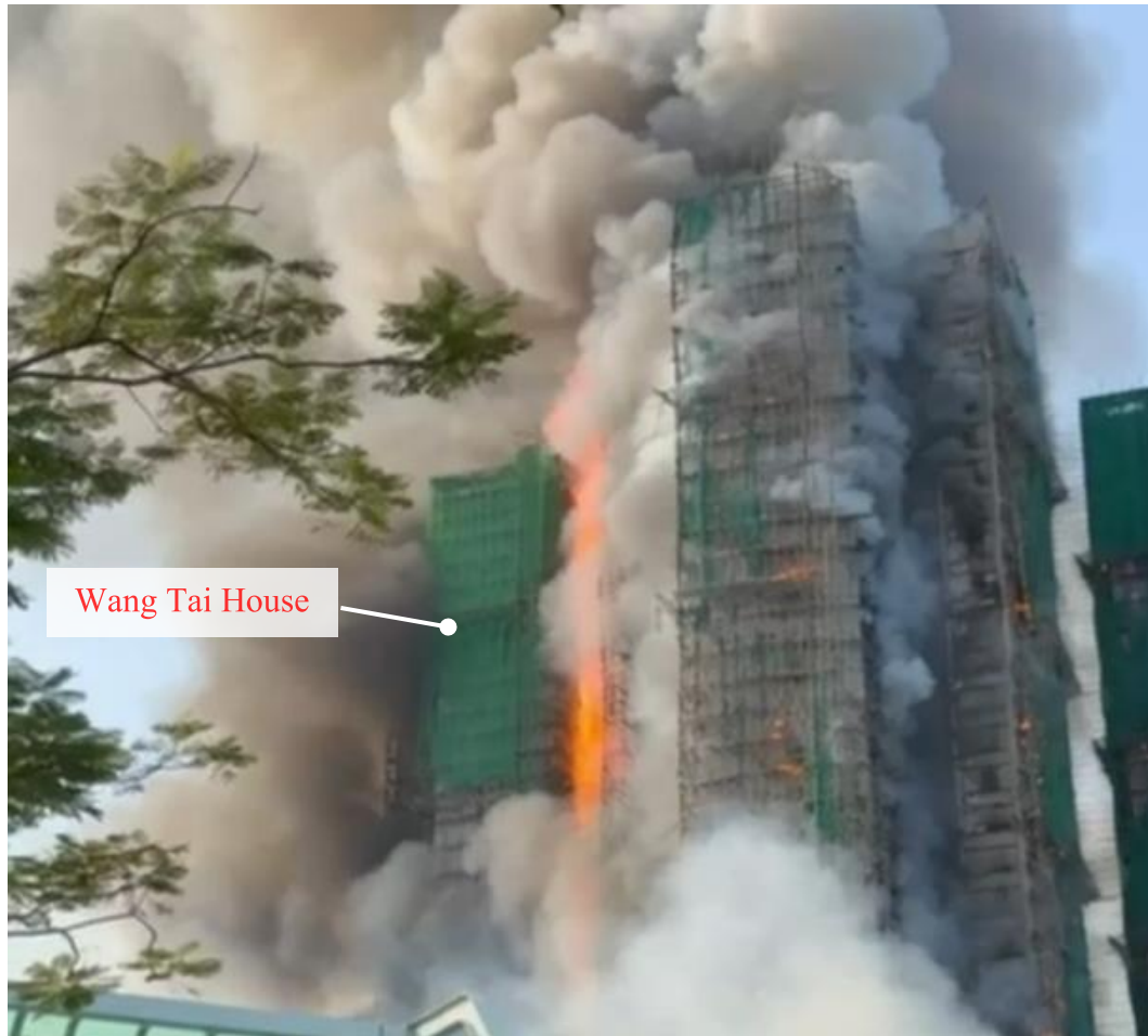
Photo 7-4: Rapid Vertical Fire Spread along the East Re-entrant of Wang Tai House at 1516 hours
