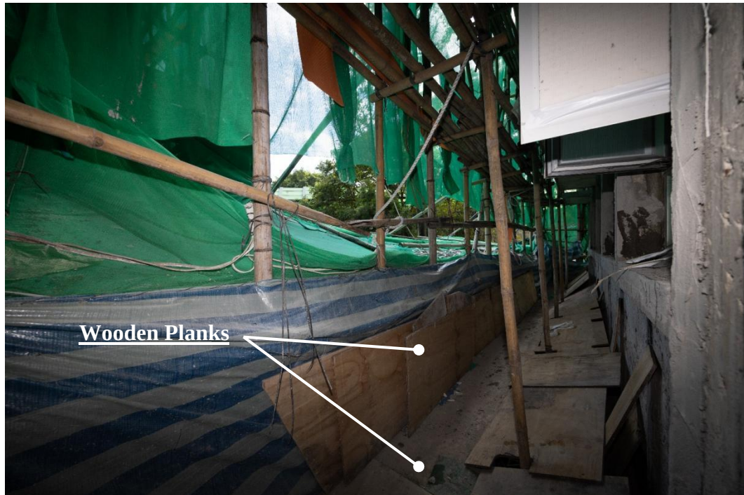
Photo 4-7: Close-up View of the Working Platforms
