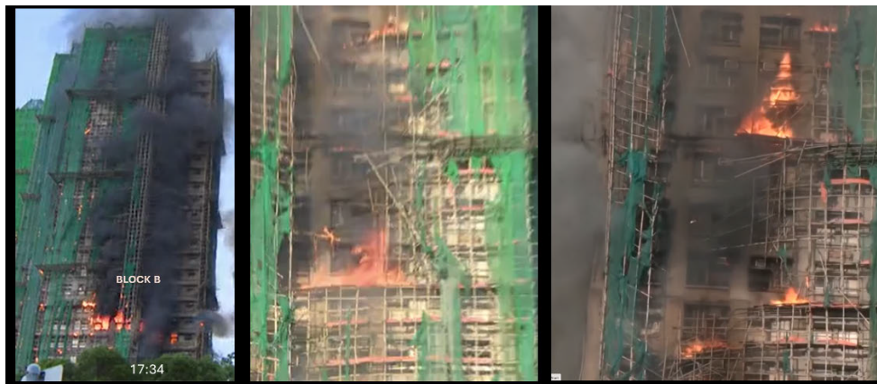
Figure 3-14. Remaining scaffolding to fuel the subsequent fire spread
