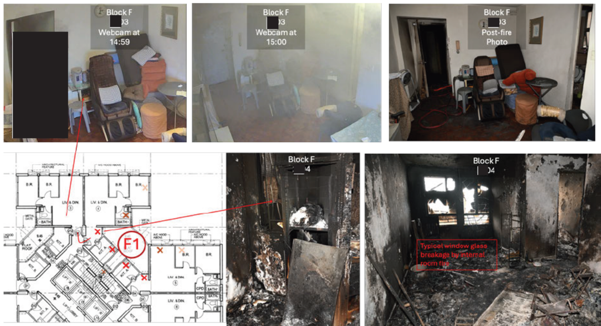
Figure 4.11. Conditions in Unit 03 of Wang Cheong House
