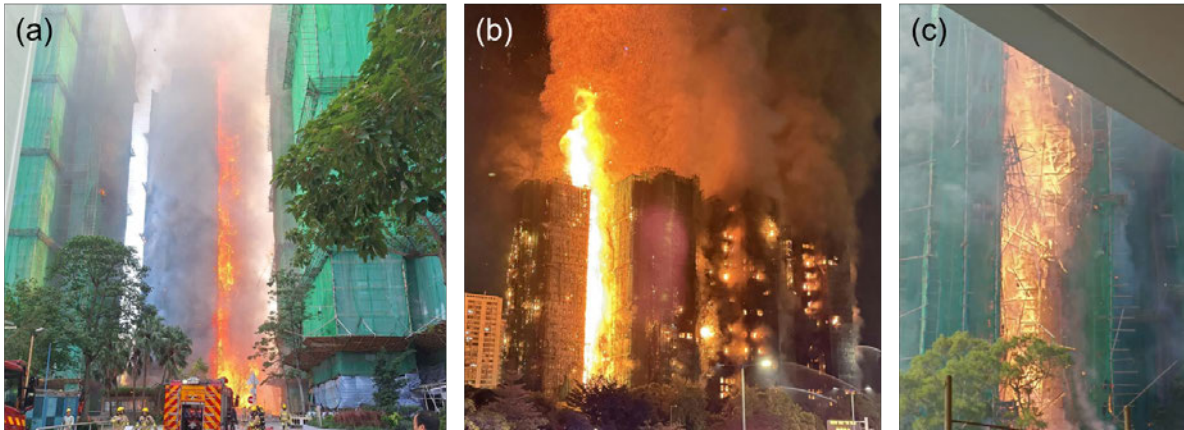
Figure 3-38. Chimney effect observed at (a) Wang Cheong House west re-entrant and (b) Wang Yan House south re-entrant, and (c) combustible scaffolding burning along the re-entrant
