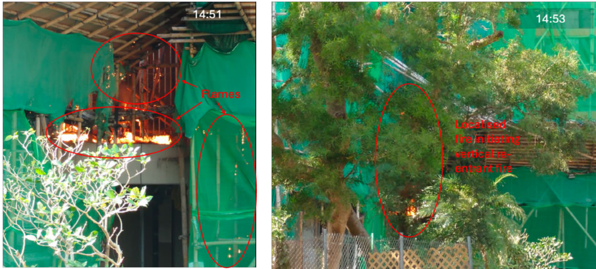
Figure 3-1. Initial fire development at re-entrant of Block F
