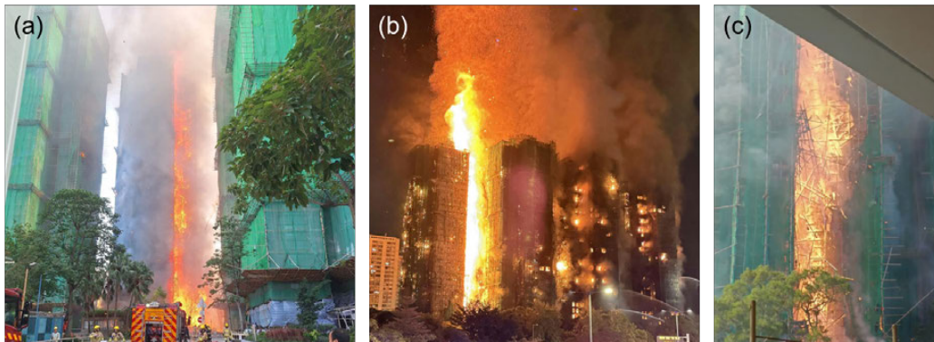
Figure 2. Chimney effect observed at (a) Wang Cheong House west re-entrant and (b) Wang Yan House south re-entrant, and (c) combustible scaffolding burning along the re-entrant (credit to RTHK and HK01).
