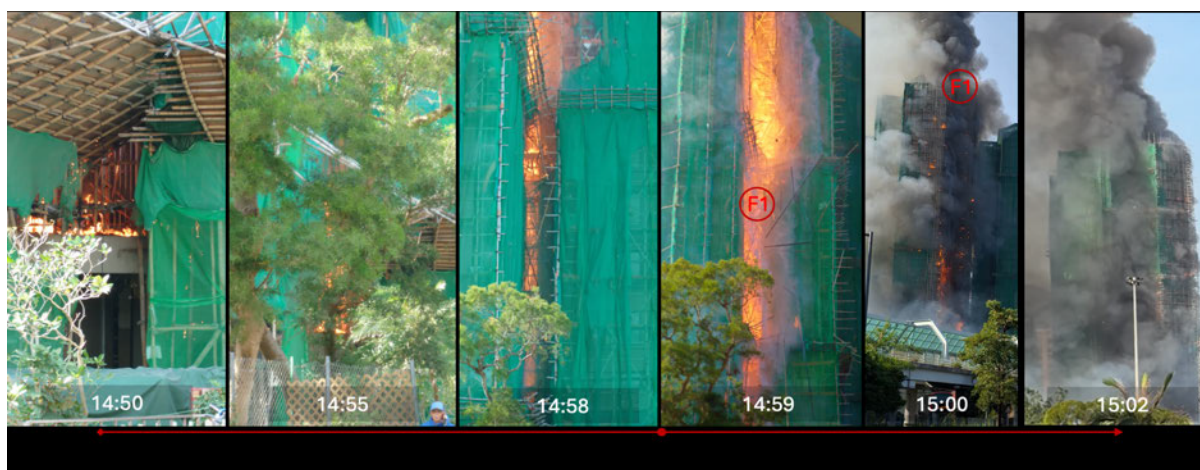
Figure 3-4. Initiation and development of F1 re-entrant vertical fire
