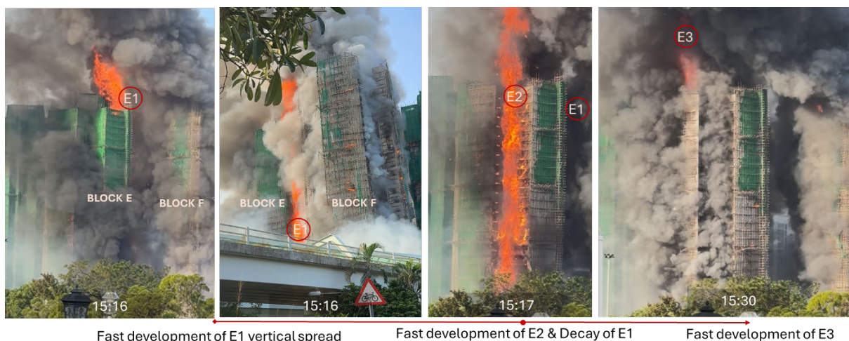
Figure 3-7. Initiation and development of E1, E2, and E3 re-entrant vertical fire
