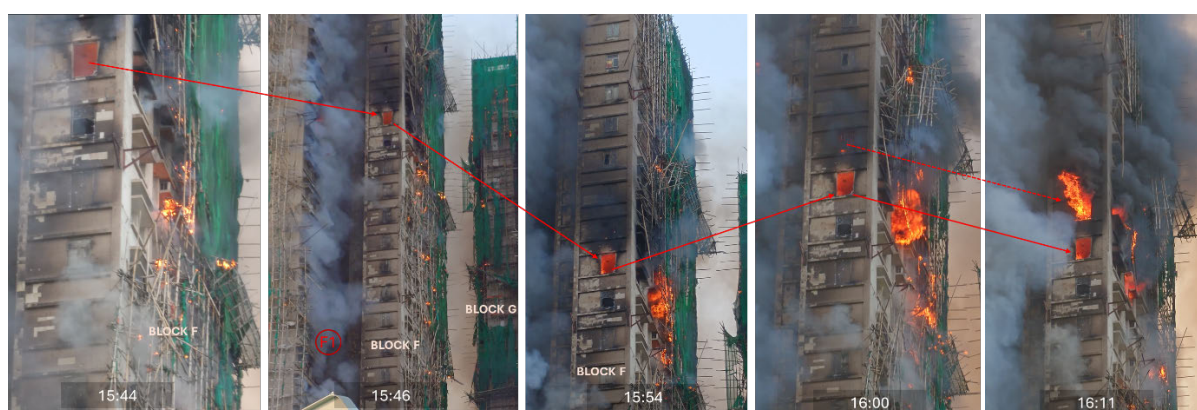
Figure 3-15. Subsequent fire spread from lower floor to upper floor
