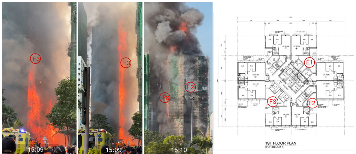
Figure 3-6. Initiation and development of F3 re-entrant vertical fire
