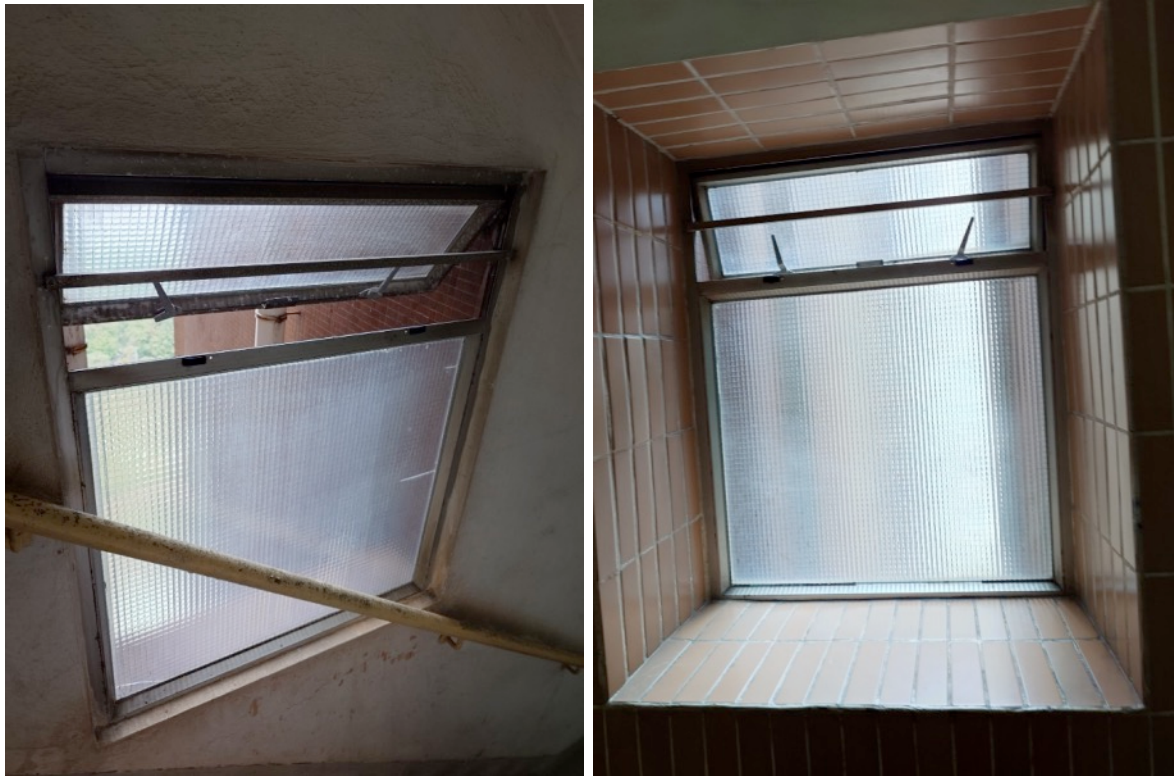
Figure 4.7. Wired glass window (WGW) in (a) staircase; (b) lift lobby
